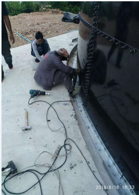
Install the base angles
