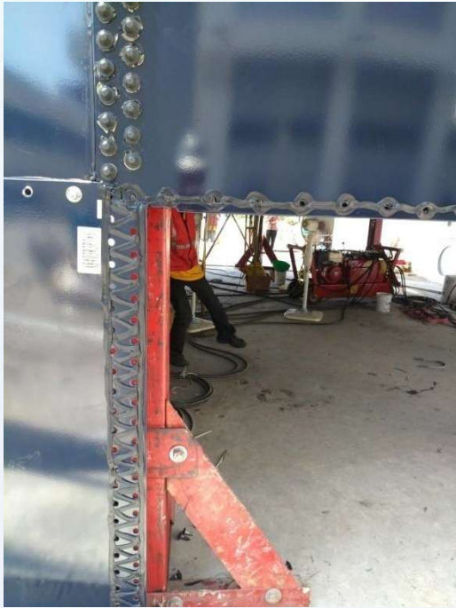
Apply the Sealant
